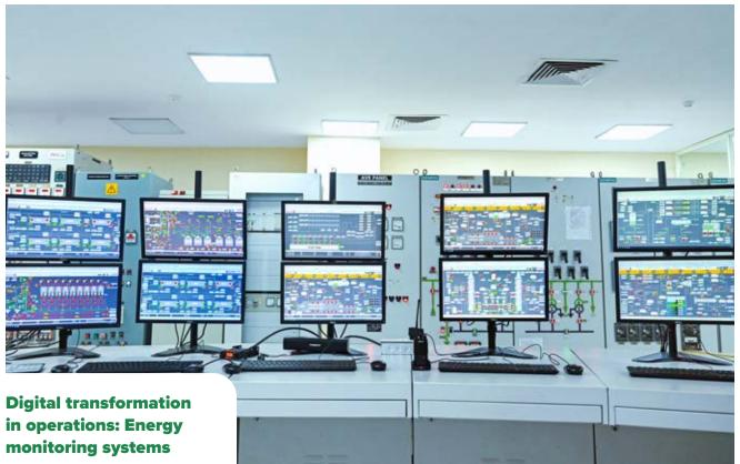
Four USA Carbon segment calcination sites completed the installation of online energy monitoring systems, providing real-time data on energy usage and breakdowns. This digitalisation initiative enables us to quantify the impact of energy reduction projects, with an anticipated total energy use reduction of over 10% in the next three years.
